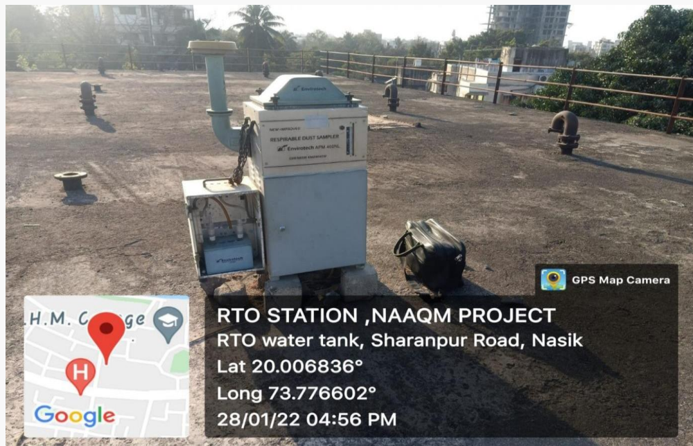
RTO Residential Air Quality Monitoring Station Colony, Pandit Colony Nashik
